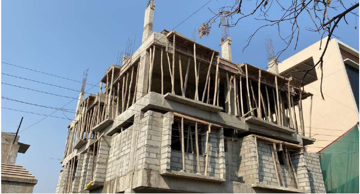
Fig: Exterior view
