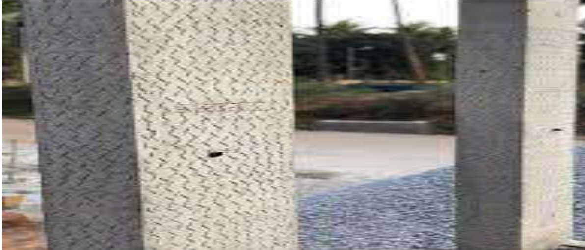
Fig: Hacking of Column
